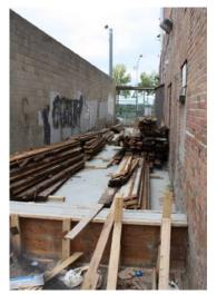
The ground floor of the eastern extension of the building has now been poured. It is currently acting as a storage space for the floor joists.
