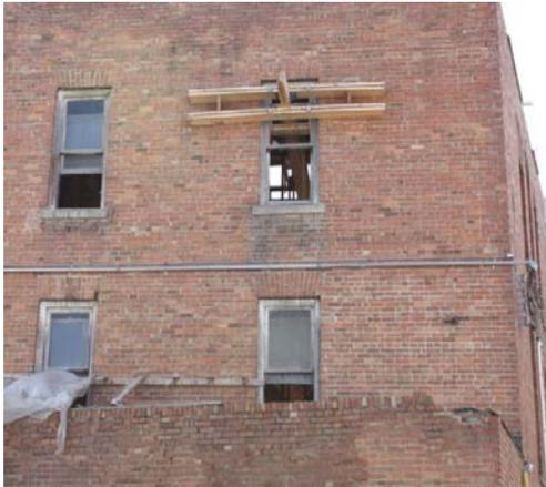
The bracing of the historic brick walls continues as more of the original support material is removed. This month a large I beam that will not be used in the new structure was cut from basement foundations. I found the bracing of the east and central walls through two third floor window openings particularly interesting.
