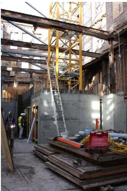
Interior concrete walls have also begun to be poured in the basement giving us a better visual picture of how the space will appear. For many of us studying a blueprint does not adequately allow us to visualize the space in three dimensions.
