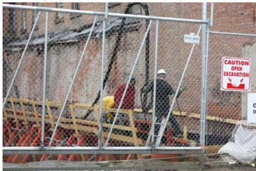
that the basement wall of the adjoining Brighton Block also had to be braced so that the pressure of the newly poured concrete would not blow out that wall causing it to collapse.
