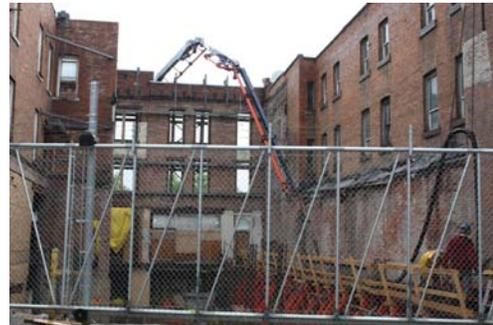
The windows on the brick façade facing Jasper Avenue have been removed to reduce the stress on the wall caused by wind. Although thoroughly braced by steel beams, this wall is essentially free standing until the new steel framework is installed this fall.
